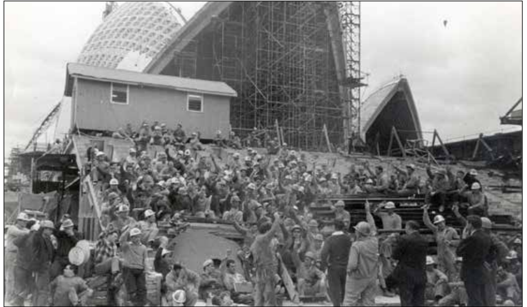
Above: Members of the BLF on the Opera House construction site in the 1960s
