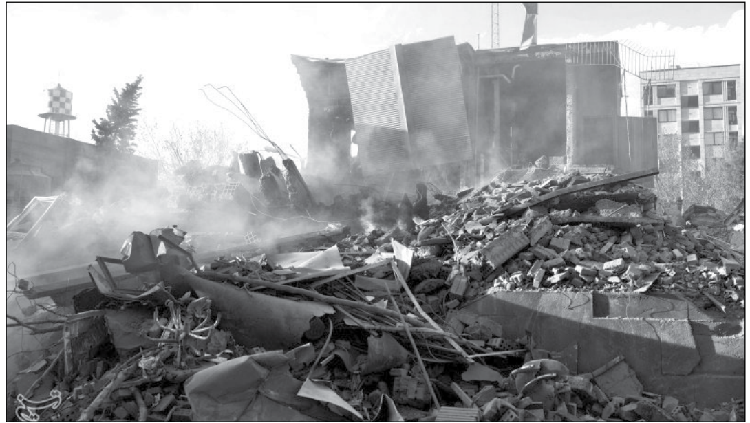
Above: Damage from an airstrike targeting the University of Science and Technology in Tehran Photo: Tasmin News Agency/Masoud Shahrestani
