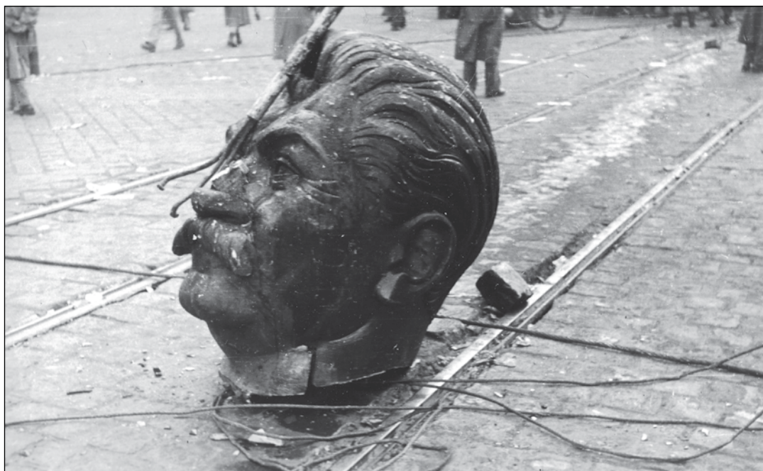
Above: Stalin's head torn off a statue and dumped on the road in Budapest during the uprising in 1956
